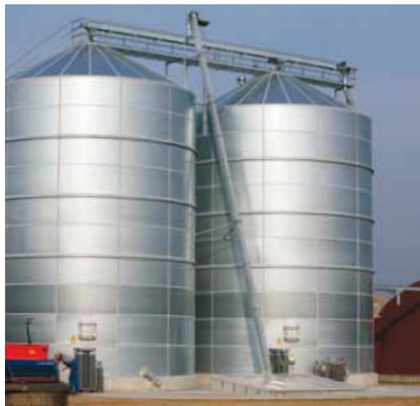
Two 930/10 silos, total 1732 m 3 . 40 tons conveyors with pit, chain elevator and walkway with reversible chain conveyor.
